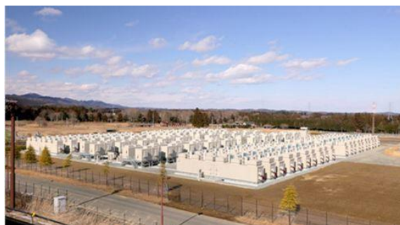
Picture of the 40 MW and 40 MWh energy storage system in Fukushima, Japan.
