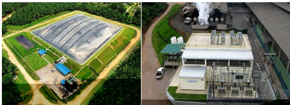
Covered lagoon type – biogas power plant of PT REA Kaltim Plantations (ref. 10)
